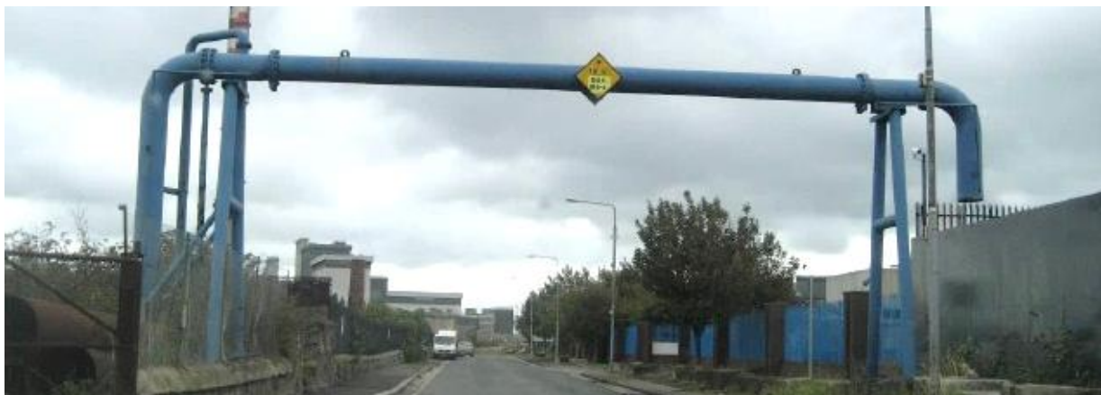
Figure 13-22: Height restriction on Pigeon House Road (6 m)
