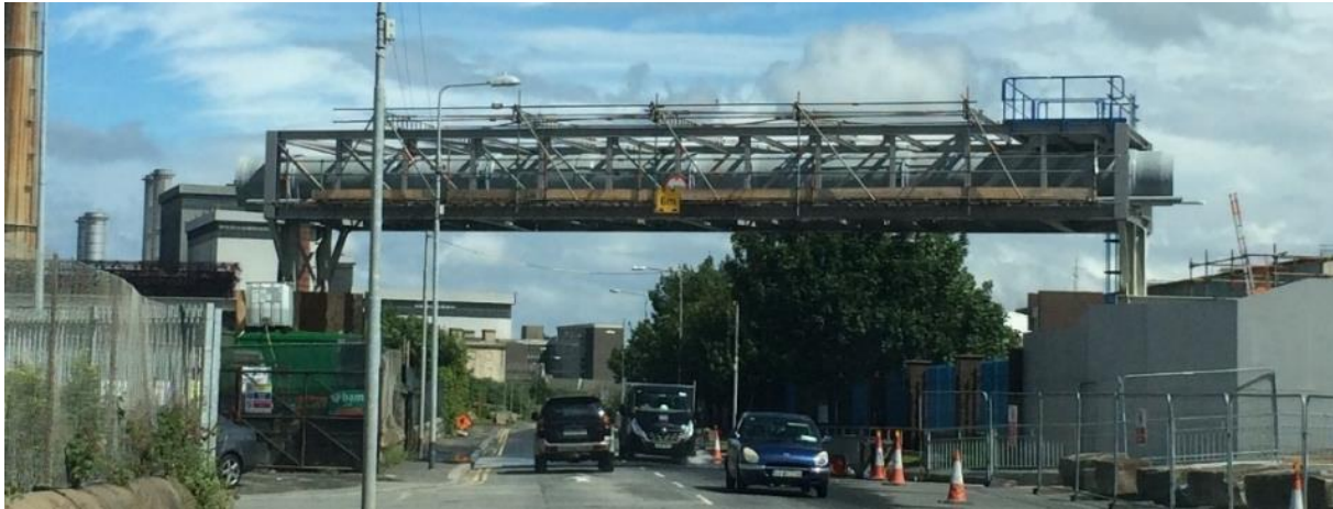
Figure 13-23: Height restriction on Pigeon House Road (6 m)
