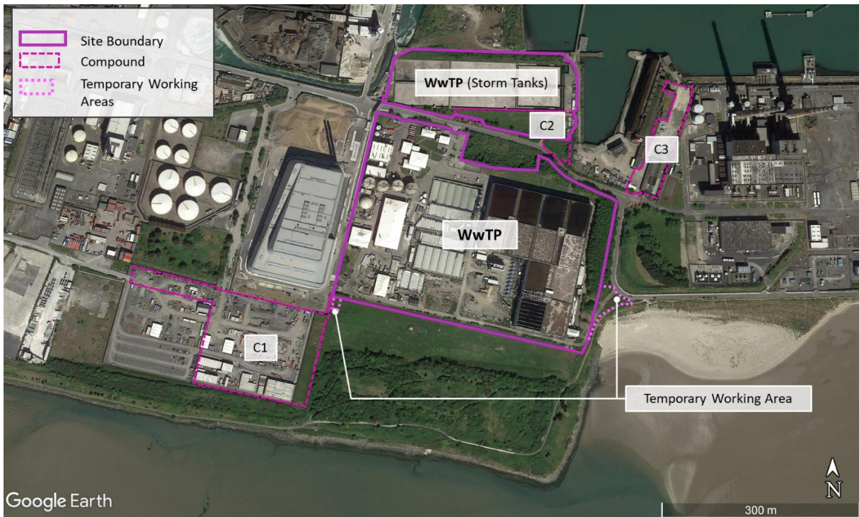
Figure 12-11: Ringsend WwTP site location
