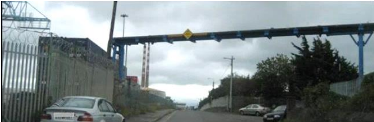
Figure 13-21: Height restriction on Pigeon House Road (5.64 m)
