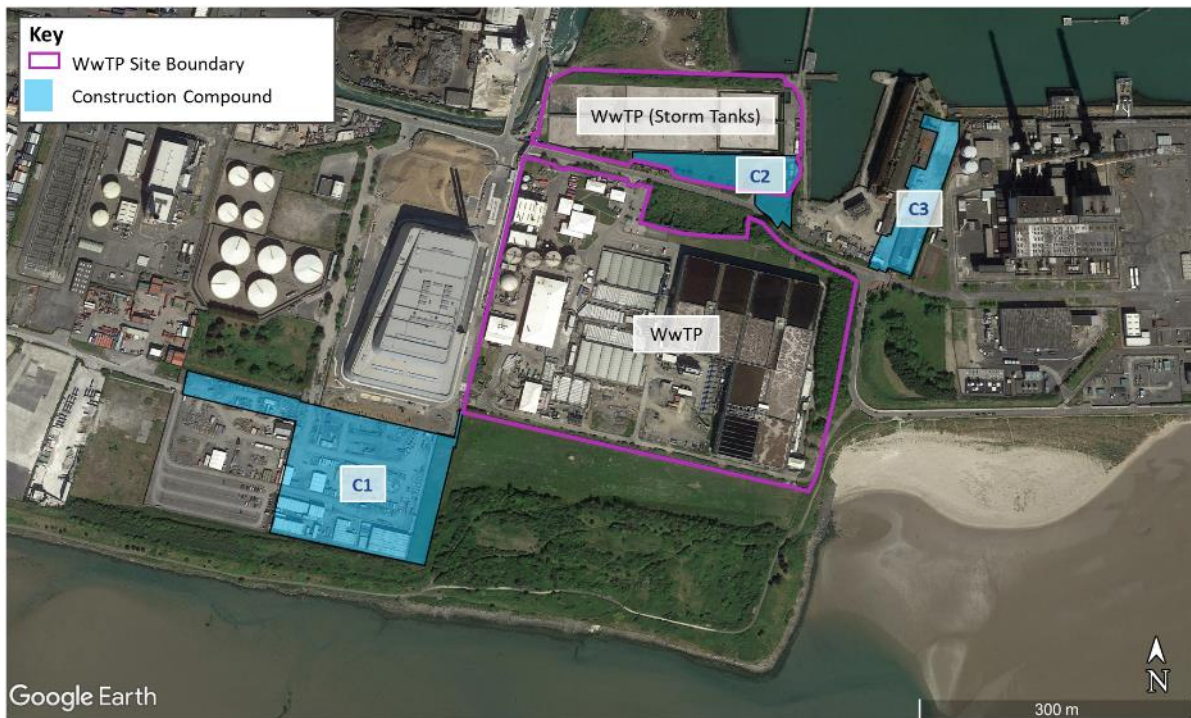
Figure 7-5: Construction Compound Areas
