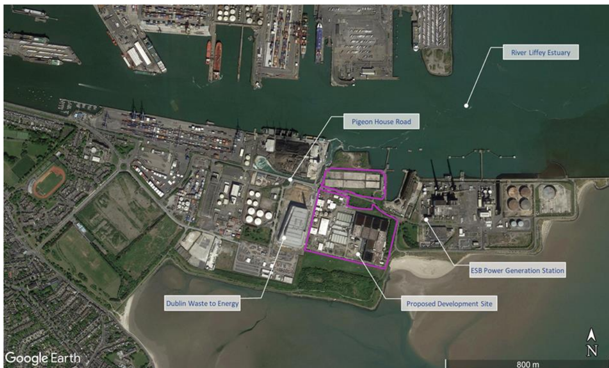
Figure 1-8: Ringsend wastewater treatment plant location
