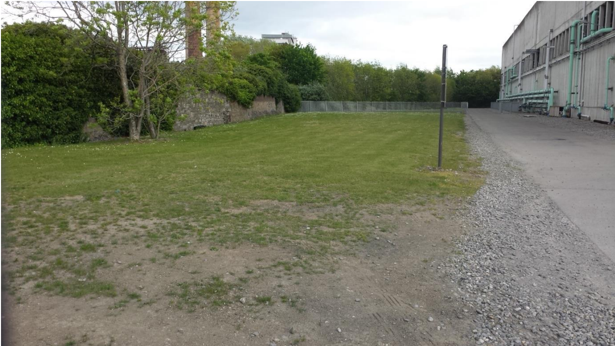
Figure 11-6: View of the south wall of the Pigeon House Fort where it faces the Ringsend WwTP site
