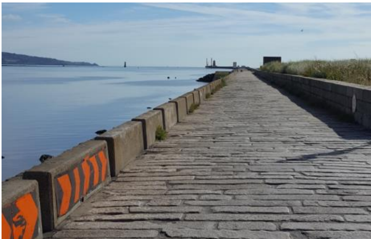
Figure 12-4: Great South Wall
