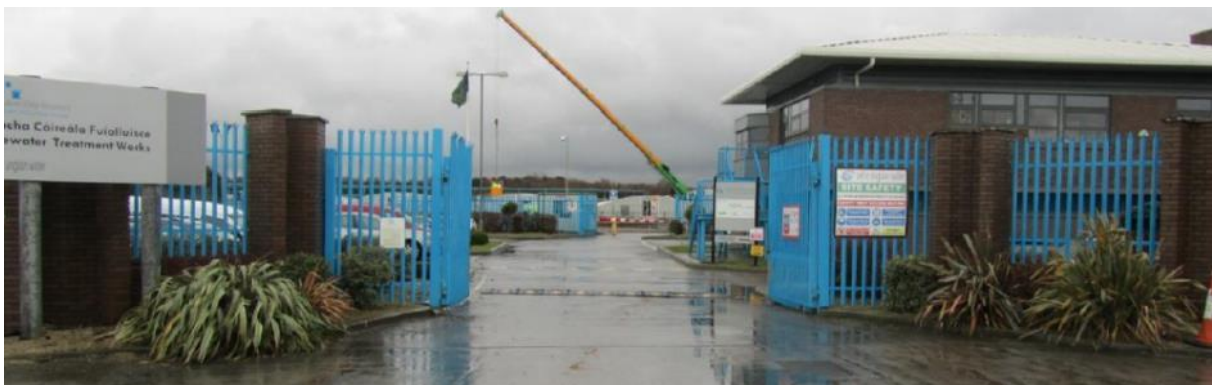
Figure 13-24: Existing WwTP Site Primary Entrance
